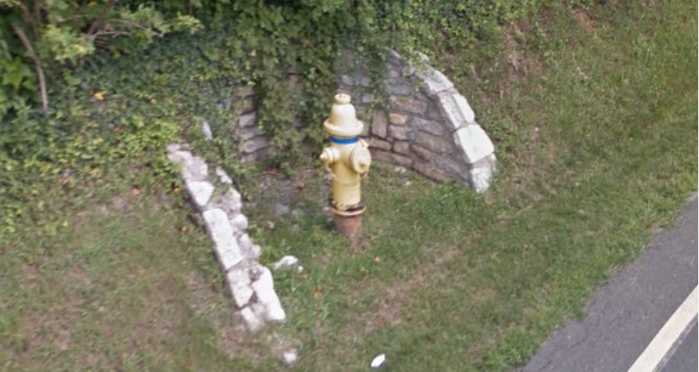
Standard stone retaining wall in Amberley Village.
