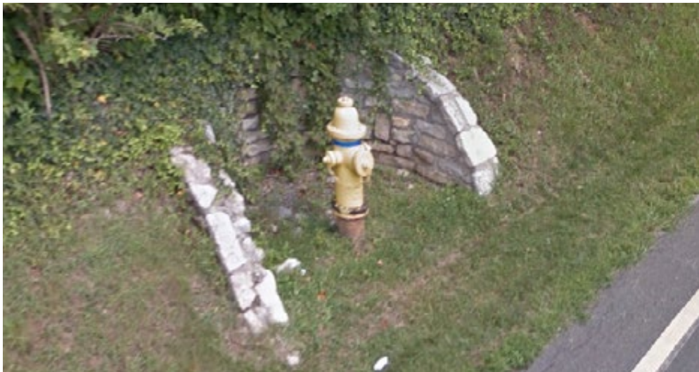
Standard stone retaining wall in Amberley Village.
