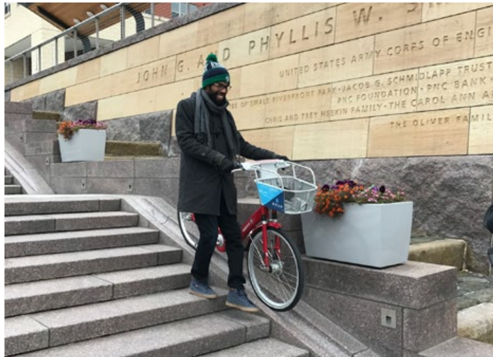
PAVED STAIRS WITH RUNNEL
