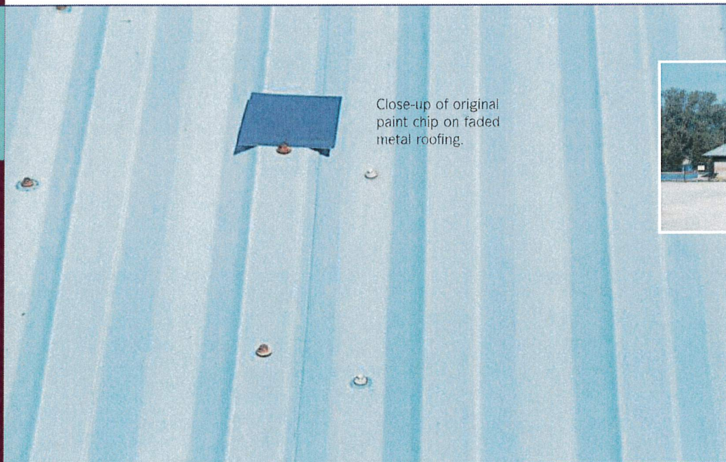
Competitive SMP coating on building after ten years in Ohio weather.
