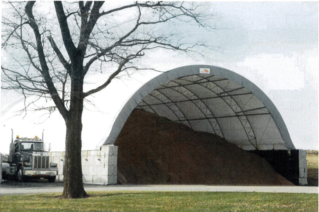
Hoop Barn on Concrete Blocks
