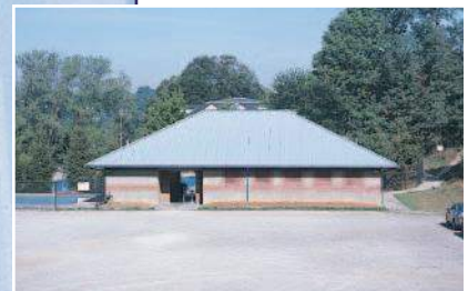
Competitive SMP coating on building after ten years in Ohio weather.
