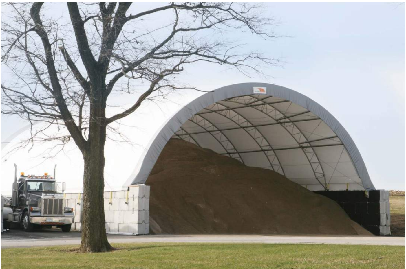
Hoop Barn on Concrete Blocks
