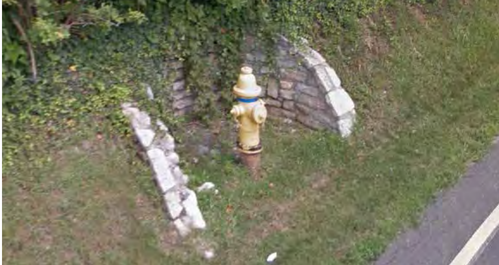
Standard stone retaining wall in Amberley Village.
