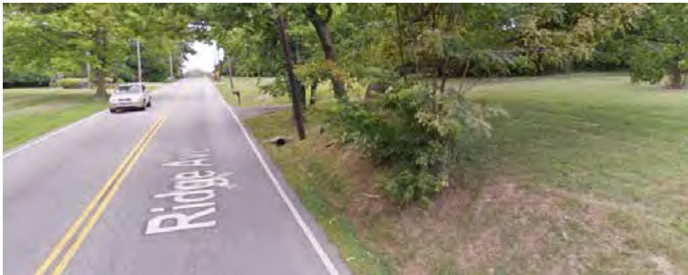
Modest Slope: In this condition the adjacent slope could be graded out and replanted to maintain the pre-existing character.
