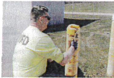
Repainting poles at the North Site
