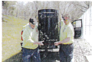
Installation of new trash cans
