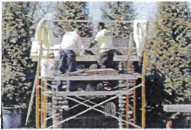
Replacing shingles at Fair Oaks
