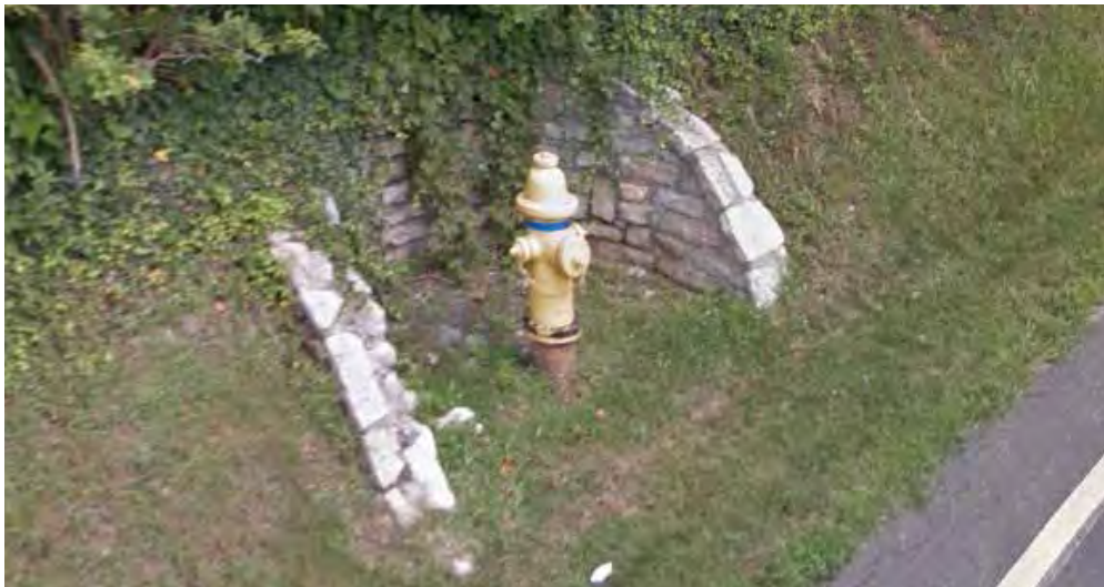
Standard stone retaining wall in Amberley Village.
